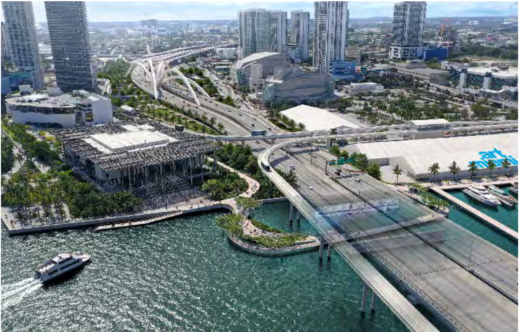
Miami DDA Pedestrian Bridge
