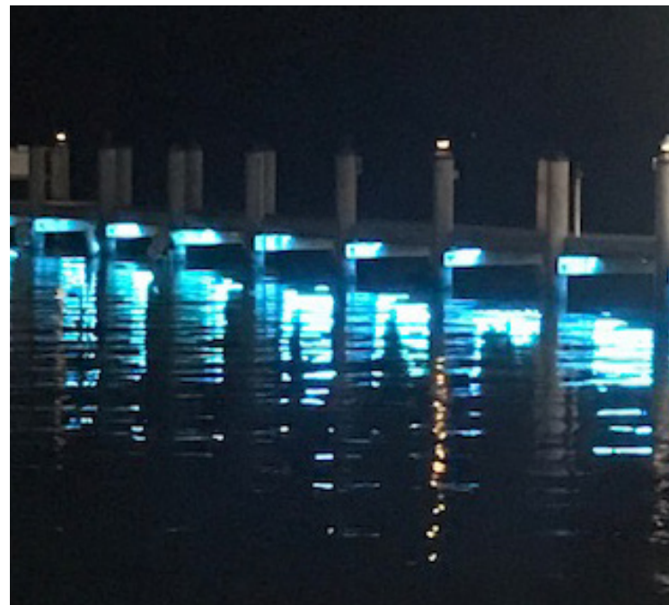
Underwater Fish Lights - for specialty locations along the water's edge
